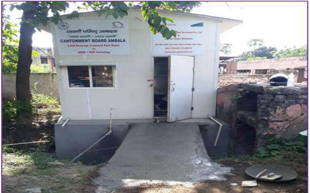
5KLD STP, CBA Office, Ambala.
